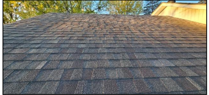
2. Asphalt shingles
