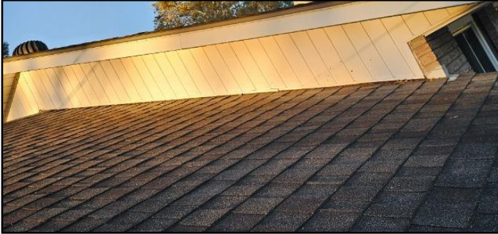
1. Asphalt shingles
