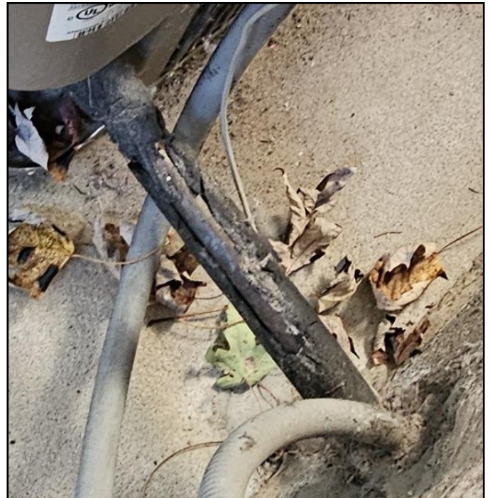
49. Insulation - missing
