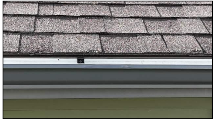
2. Asphalt shingles
