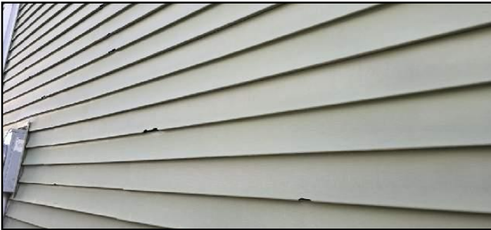
24. Mechanical damage
