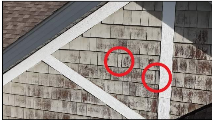
28. Mechanical damage
