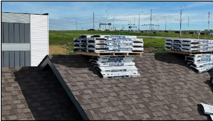
1. Asphalt shingles
