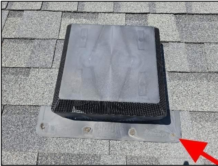
2. Exposed fasteners
