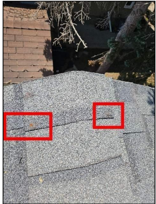
3. Exposed fasteners
