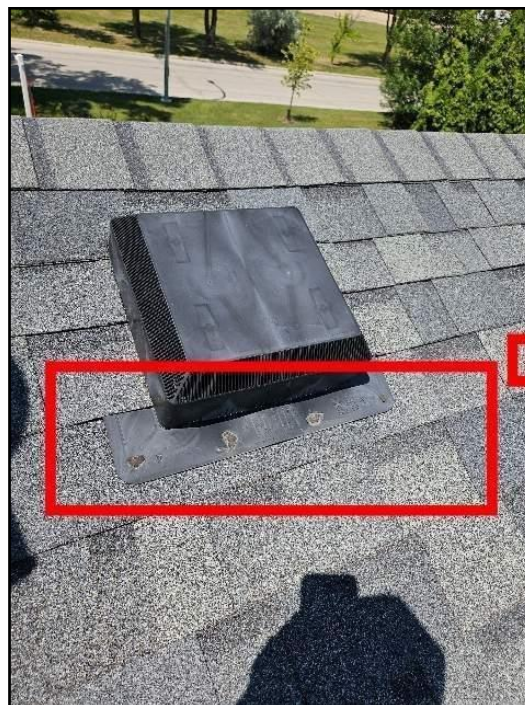
4. Exposed fasteners
